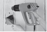
• Using a heat gun at temperatures greater than 1100°F.
